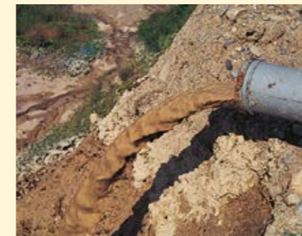
Removing slurry from a tunnel
